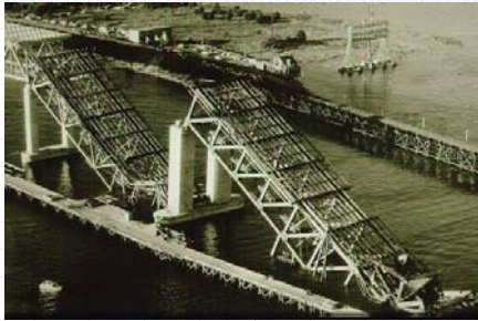
Oops: Collapse of the Second Narrows Bridge, Vancouver
