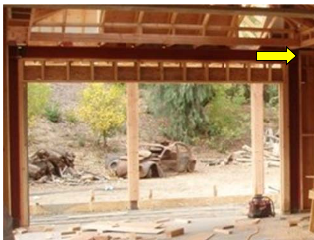
Figure 10: Applied earthquake load on the moment frame
