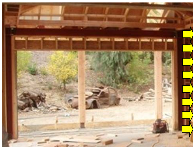
Figure 9: Applied wind load on the moment frame
