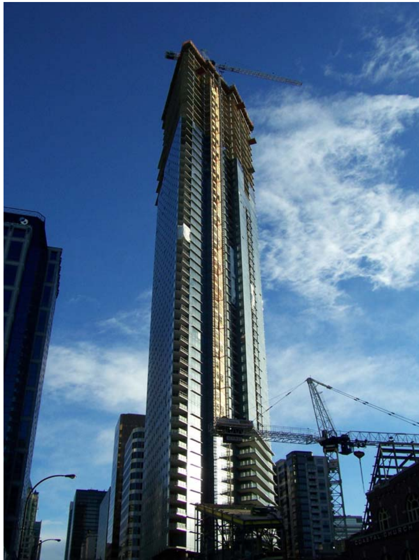
Living Shangri-La during construction, January 2008 (photo by Jake Plut)
